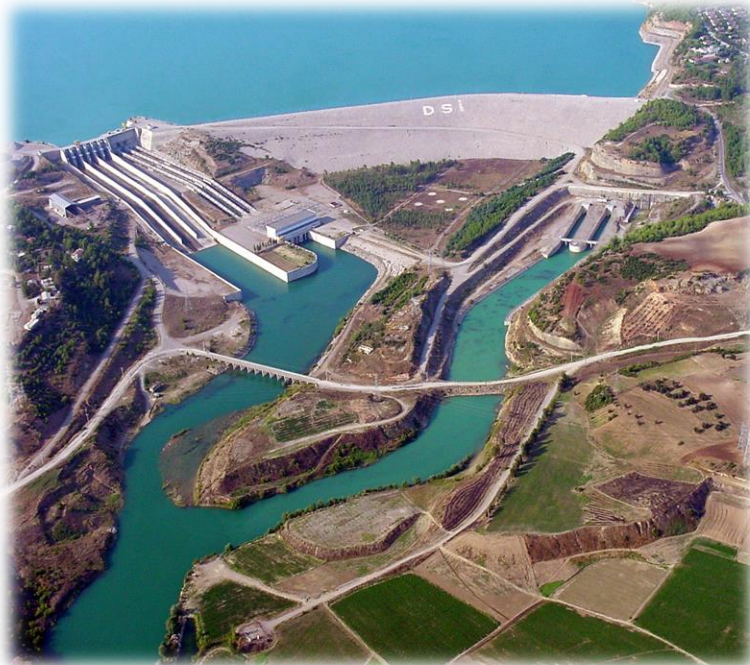
ÇATALAN HYDROELECTRIC POWER PLANT
